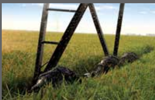
Three-Wheel Tower Structure
